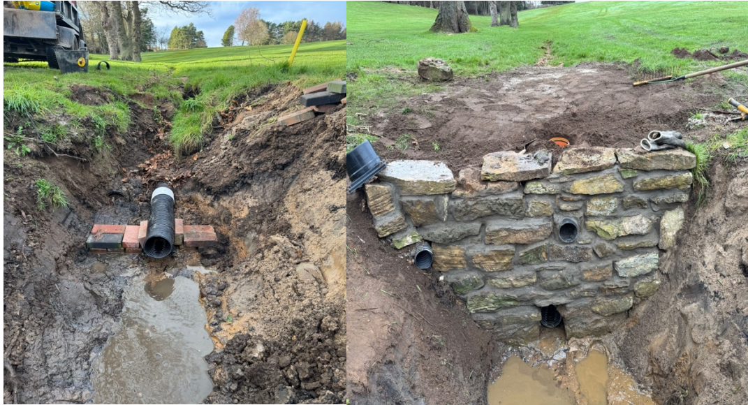
Figure 5: Drainage pipe before (left) and after, with newly constructed wall (right)
