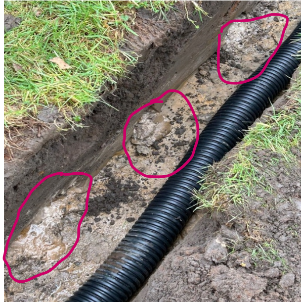
Figure 2: Running sand highlighted in the red
